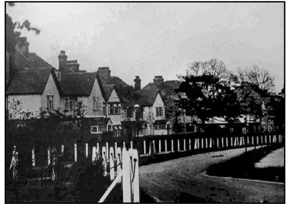
Original chain link fences.
