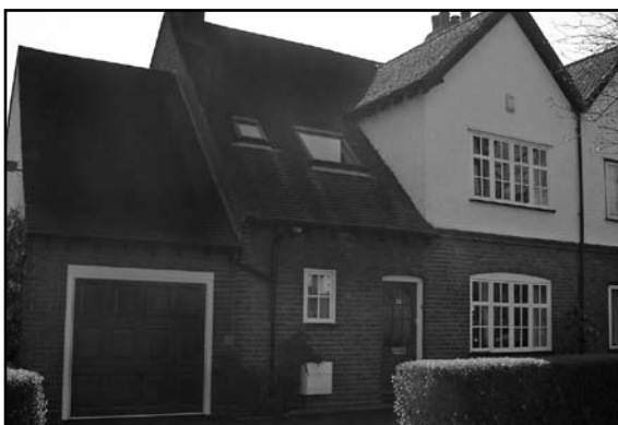
Non original skylight.
