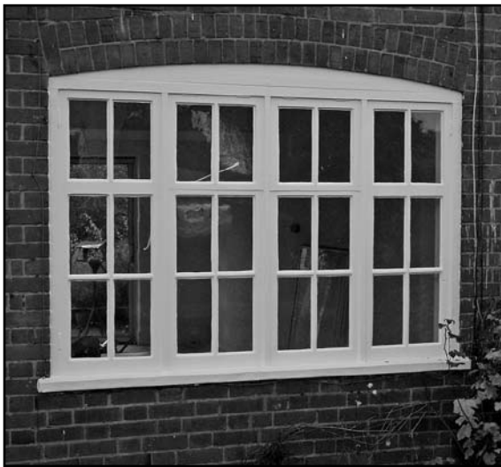
Original window recently repainted.
