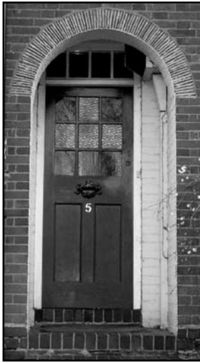
Original nine panel front door with an original door knocker.
