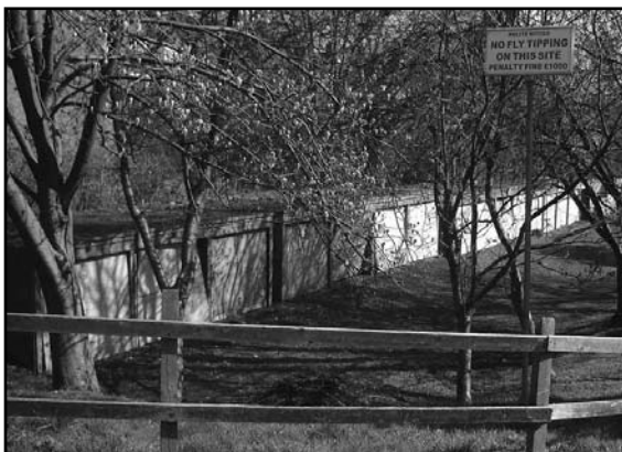
Garages on the valley site.
