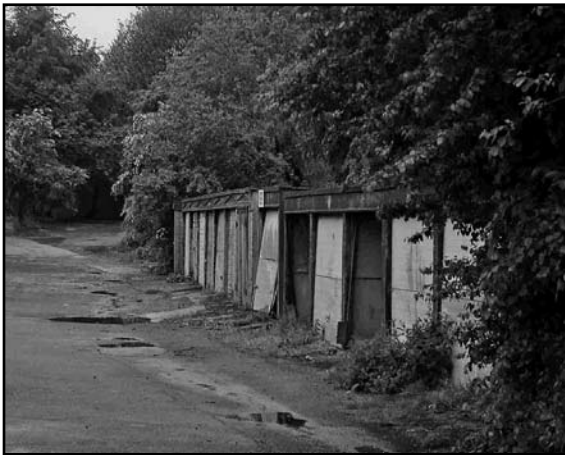
Garages on the Valley site.
