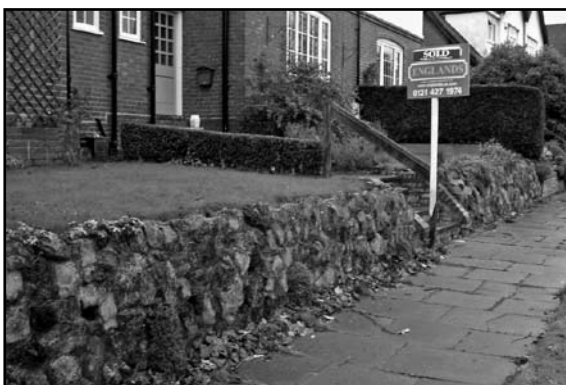
A cemented garden wall.
