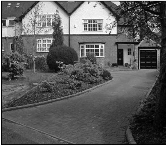
Traditional boundaries removed for block paving, Carless Avenue.
