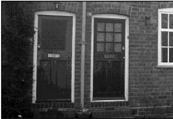
Original doors, with and without glazing bars.
