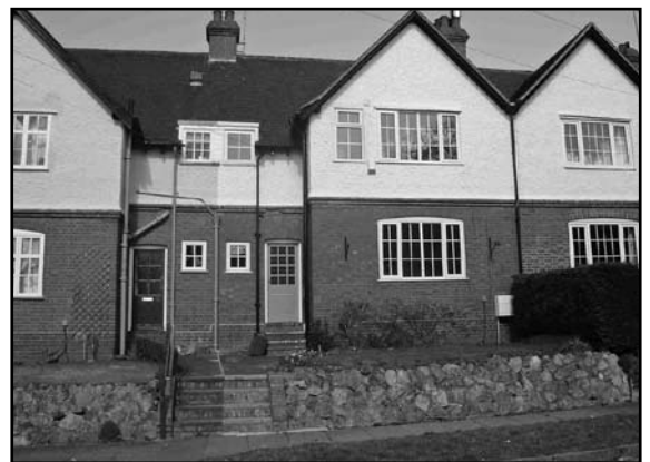
Existing original wall.
